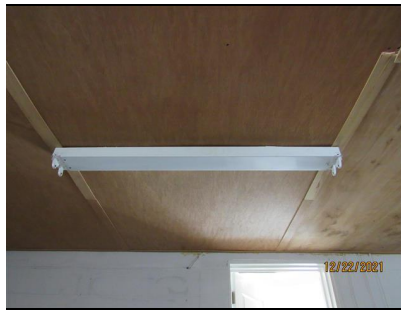
8.3 Item 1(Picture) Garage
