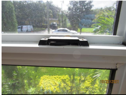
5.5 Item 3(Picture) Front Corner Bedroom
