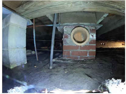
Remnant of old chimney
